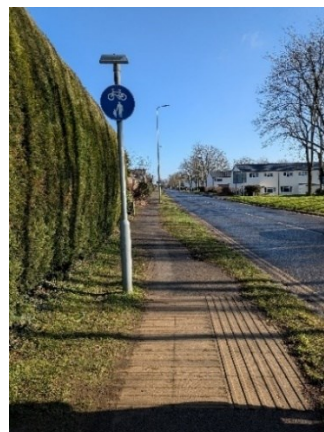
Figure 64: Unclear/ incorrect signage and tactile paving indicating a shared use footway/ cycleway
