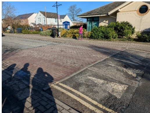
Figure 73: Raised speed hump not clear if it is to be used as a pedestrian priority crossing due to surface
