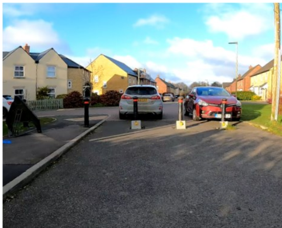
Figure 89: Modal filter at the northern end of Swinbrook Road
