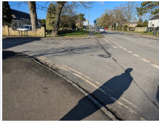
Figure 72: Missing tactile paving on dropped kerbs when crossing Rock Road along Burford Road
