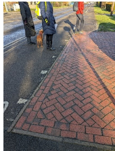
Figure 82: Some driveways extend out into the shared use footway/ cycleway
