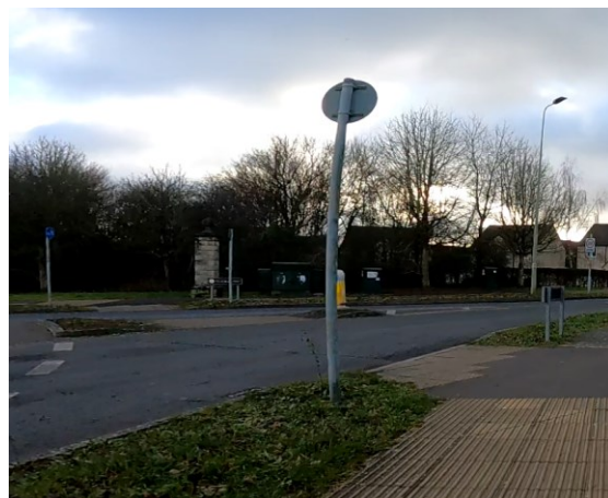
Figure 104: The shared use footway/ cycleway does not have priority over road vehicles at side-roads
