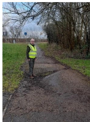
Figure 93: The surface has lowered, exposing some raised ironworks, making the surface a very poor condition
