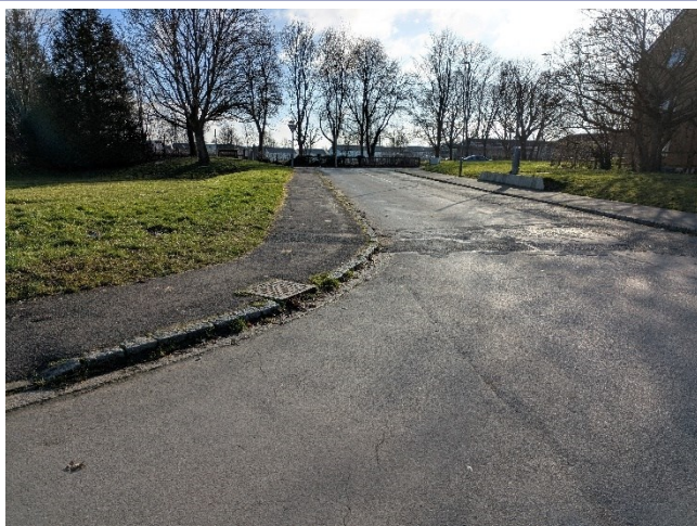
Figure 94: Missing dropped kerbs on side roads, however this land is earmarked for development in the future
