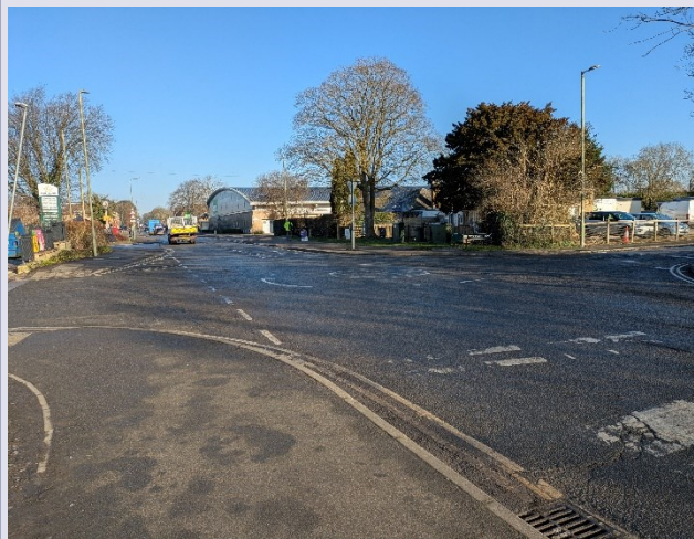
Figure 79: Mini roundabout marking faded, with pedestrian movements difficult and unsafe
