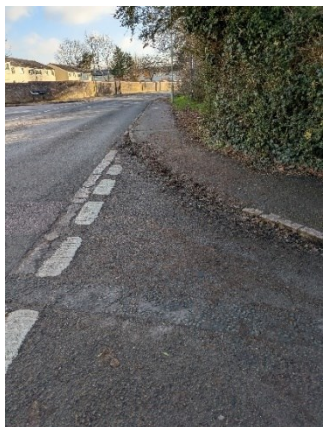
Figure 65: Missing tactile paving and unmaintained dropped kerb, with footway narrowed due to poorly maintained verge
