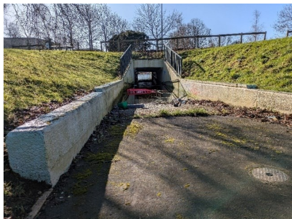
Figure 63: Underpass on eastern section of Upavon Way flooded with litter in standing water
