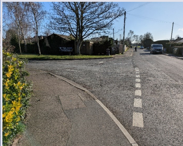
Figure 88: Junction of Swinbrook Road and Glenmore Road very wide and missing tactile paving on dropped kerbs
